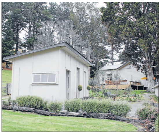
At home: The old store shed and homestead fit easily into the surrounds after renovation.
